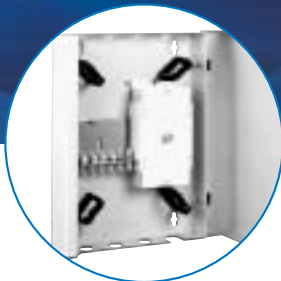
installed: 5 splice cassettes, 1 patch panel (12 ports)
